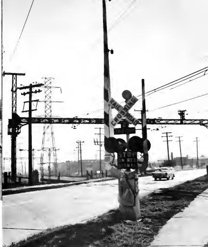
As on a main line railroad, automatic crossing gates, with interconnected motorman's signal lights, give priority to train passengers at the seven grade crossings. Rehabilitation work included installation of fifteen new gates like these at Niles Center Road.
